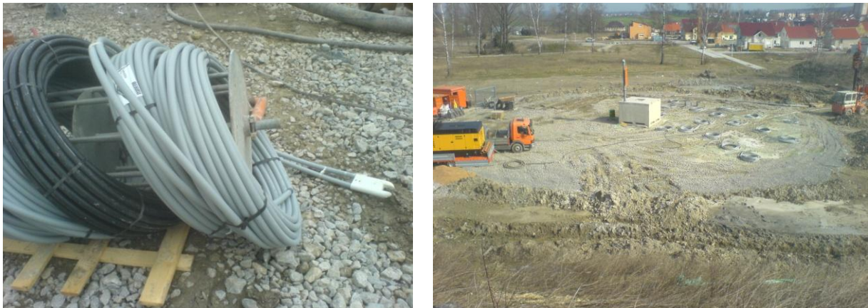
Fig. 2: BHE coils (left) and overview on the BTES construction site (right)
