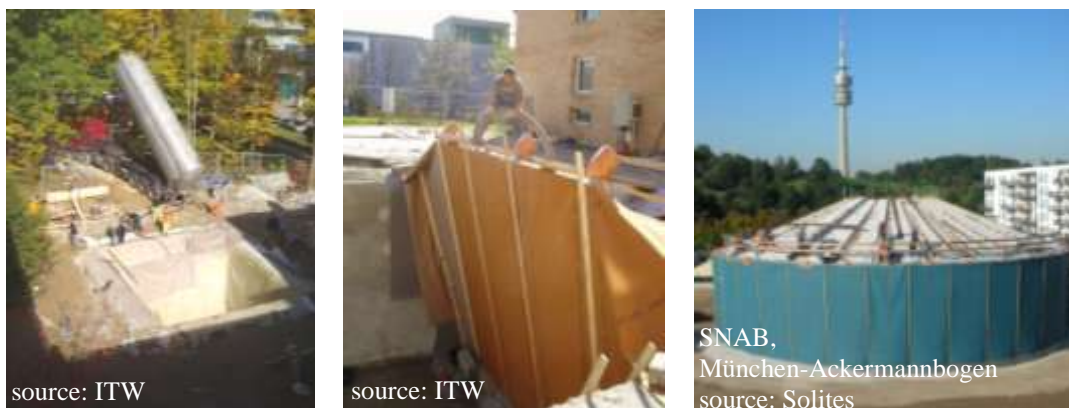
Fig. 4: Bulk insulation material in membrane-formwork with diffusible liner
