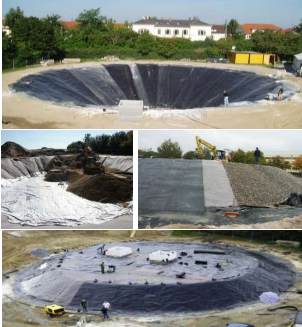
Fig. 5: Construction of the gravel-water pit TES
