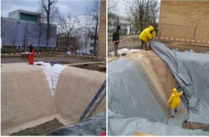
**Figure 9.** Installation of the GCL in outdoor laboratory
