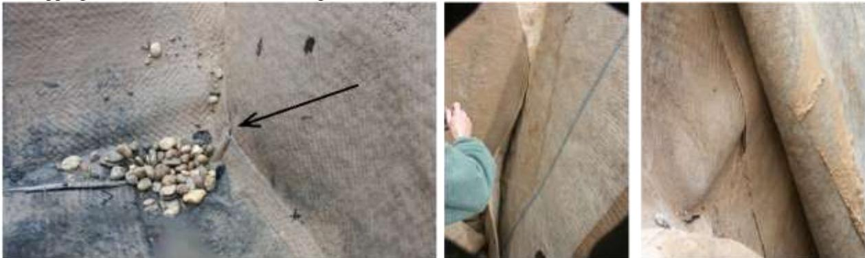
**Figure 10.** Installation errors: left: folding at the edge of the pit; centre: fabric on fabric; right, formation of a folding due to slip of the GCL
