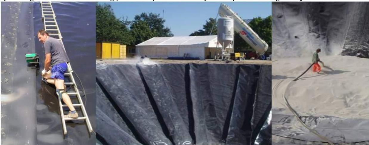
**Figure 7.** Installation of the insulation by filling loose bulk into chambers made of HDPE-barrier liners; insulation as loose bulk onto the bottom by blowing from silo-truck (gravel-water TES in Eggenstein-Leopoldshafen, ITW)
