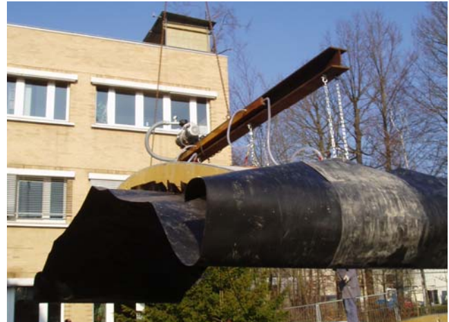
Fig. 4: Sandwich element with liner is moved by truck mounted crane
