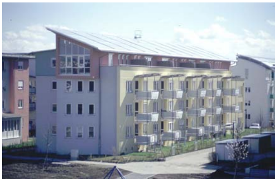
Figure 3: Roof integrated collectors on top of a multi-family building in Friedrichshafen
