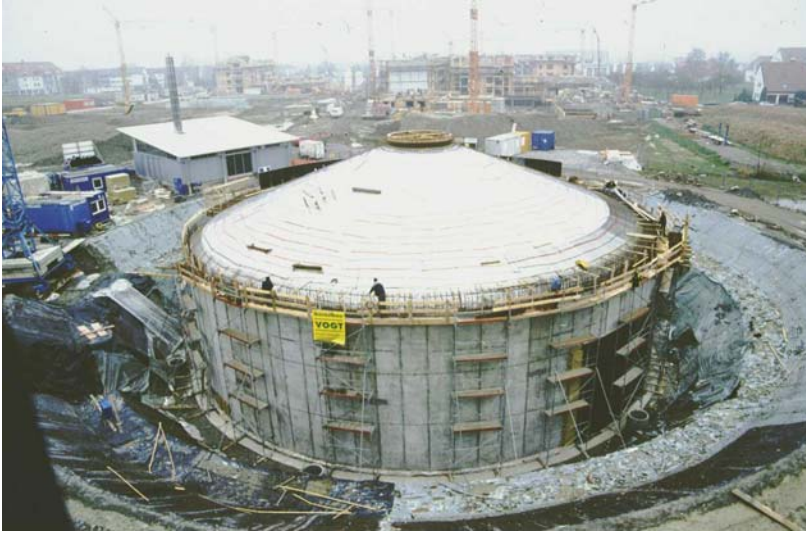
Figure 5: Hot water heat store during construction
