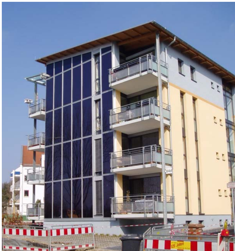
Figure 1: One of the five multi-family houses of plant C with solar thermal collector field (facade)
