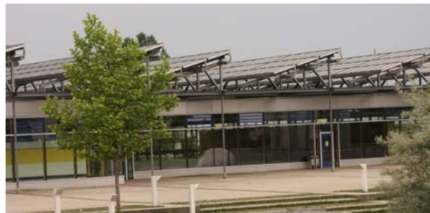
Fig. 8: Solar collectors on the gymnasium
