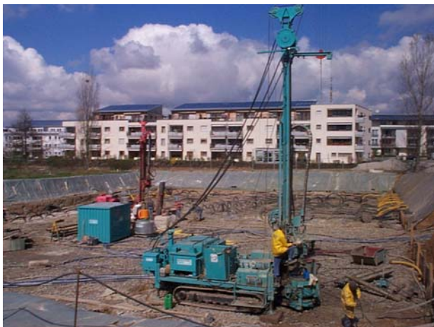
Fig. 6: Duct heat store under construction (2. extension)
