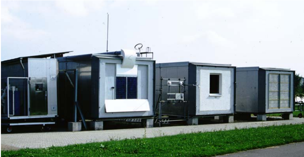
Fig. 4: South View PASSYS Test Facility at ITW
